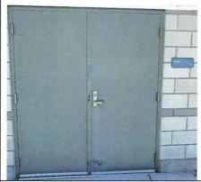
External door in Tank Room storage area public installed in 2006, replace with similar door Schlage Hardware is to be used for key replacement. Reuse open/close door magnetic door sensor and wiring.
