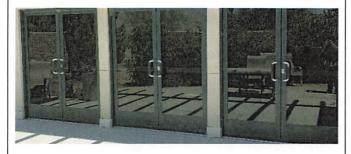
Currently three double push bar doors, installed in 2005, to be replaced with one set of push double door (middle), the other two sets replaced with windows.
