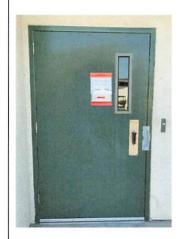
External door in public outreach area leading to fleet parking installed in 2001, replace with similar door. Doors are electronically locked through Avigilon Access Control System. Doors are normally closed to the public during the day.
