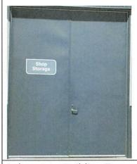
External door in storage area public installed in 2001, replace with Atlas Roll-up Door. New magnetic floor hardware will be tied into existing access control using existing wiring.
