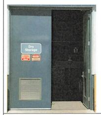
External door in storage area public installed in 2001, replace with Atlas Roll-up Door. New magnetic floor hardware will be tied into existing access control using existing wiring.
