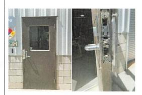
External door in Shop Welding Door installed in 2006, replace with similar door. Doors are electronically locked through Avigilon Access Control System. Doors are normally closed to the public during the day.
