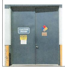
External door in storage area public installed in 2001, replace with similar door and Schlage Hardware is to be used for key replacement. Reuse open/close door magnetic door sensor and wiring.
