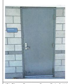
External door in Tank Room storage area public installed in 2006, replace with similar door Schlage Hardware is to be used for key replacement. Reuse open/close door magnetic door sensor and wiring.
