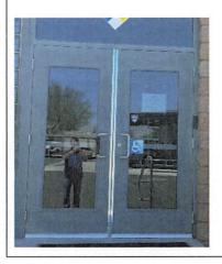
Replace entrance double doors, installed 2006, with ADA doors. Doors are electronically locked through a Avigilon Access Control System. Doors are normally open to the public during the day.
